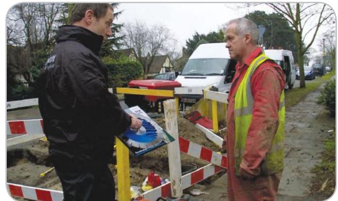
Service & support on site
